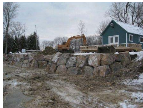
The new retaining wall during construction.
